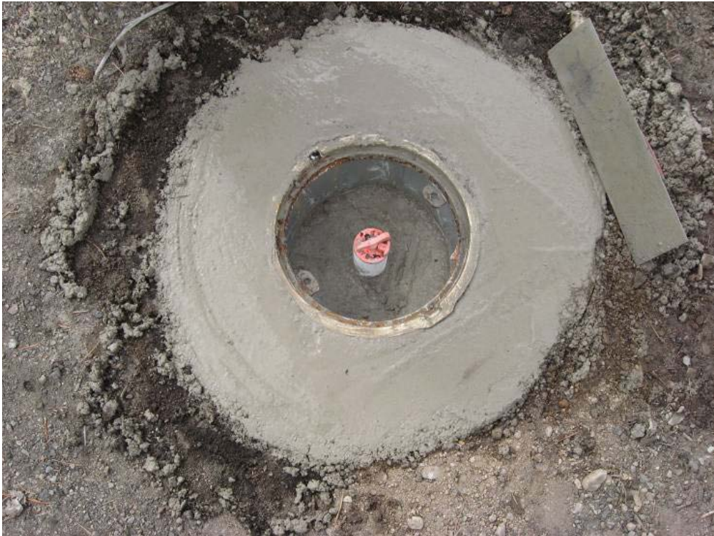
Completed PlumpJack Squaw Valley Inn Deep Well
