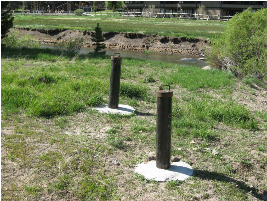
Completed Poulsen Property Wells Drilling, June 2010
