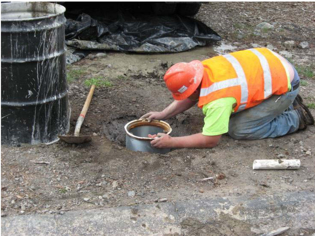
Setting Protective Casing
