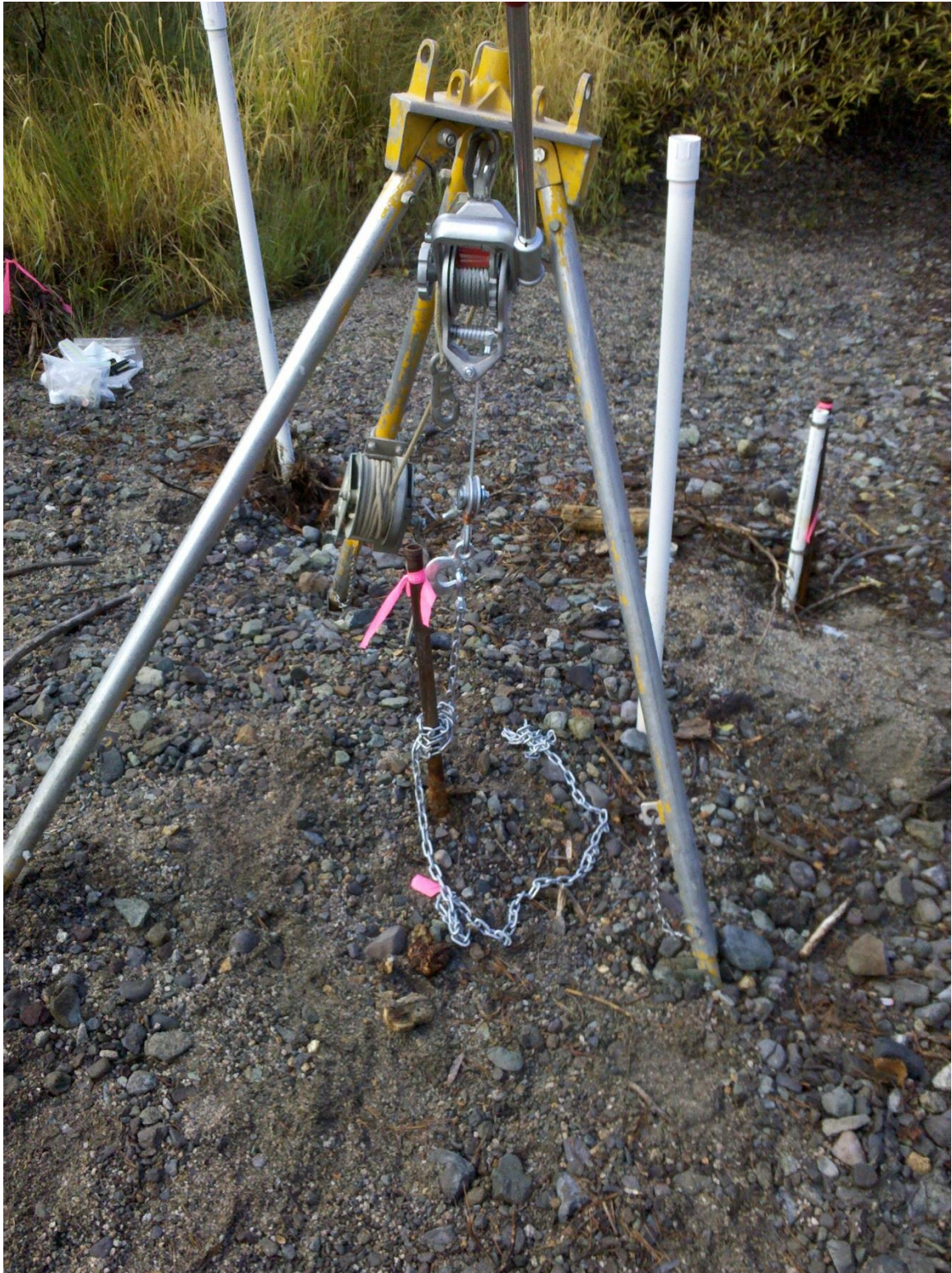
Figure A-10: Removal of Piezometer
