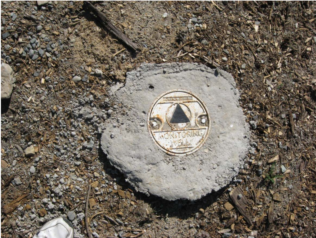
Completed PlumpJack Squaw Valley Inn Well
