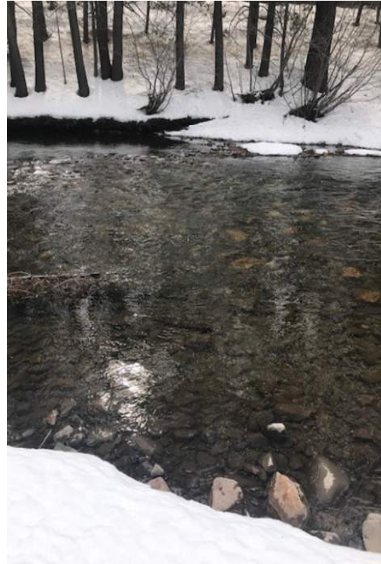
Up stream / middle view at diversion point
