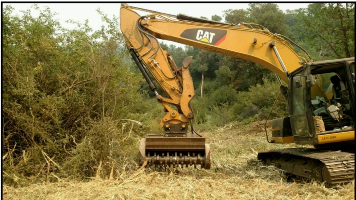
Figure 26: Excavator with masticating attachment.
