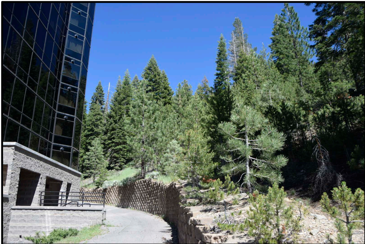
Figure 13: Pine thickets create a torching hazard adjacent to major infrastructure. This is not only a fire danger, but provides a bad example to the rest of community. This area should be heavily thinned within 150 feet of the buildings.
