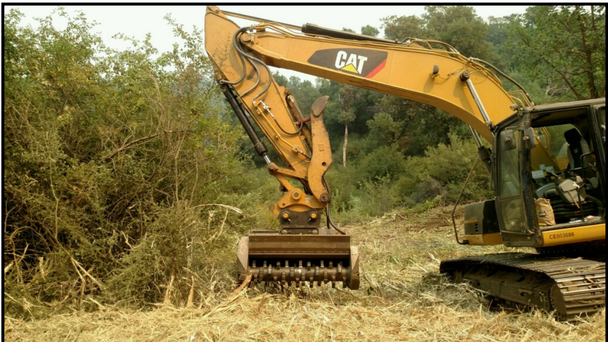
Figure 26: Excavator with masticating attachment.
