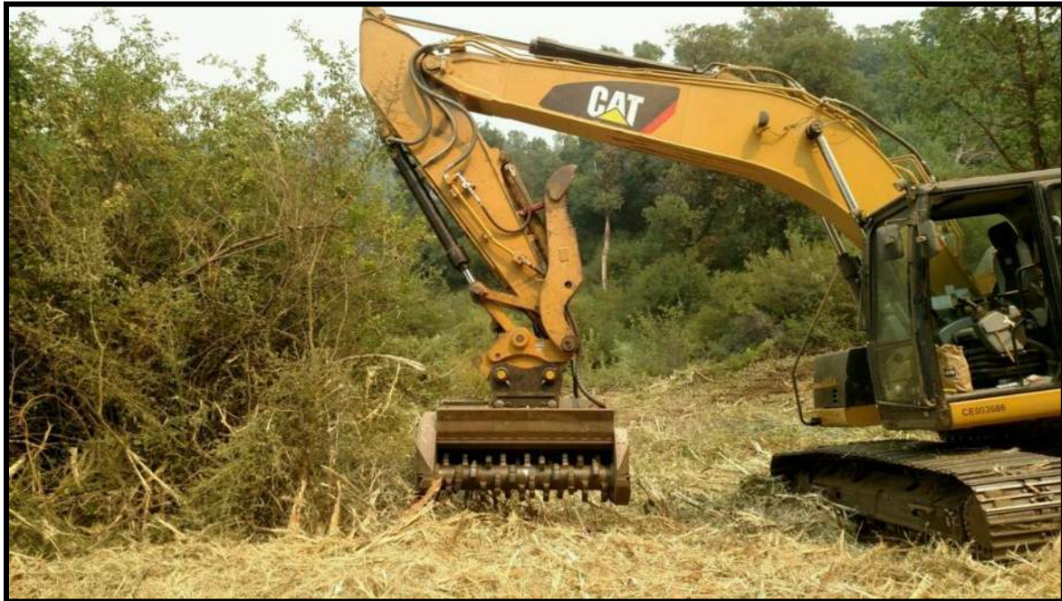
Figure 24: Excavator with masticating attachment.
