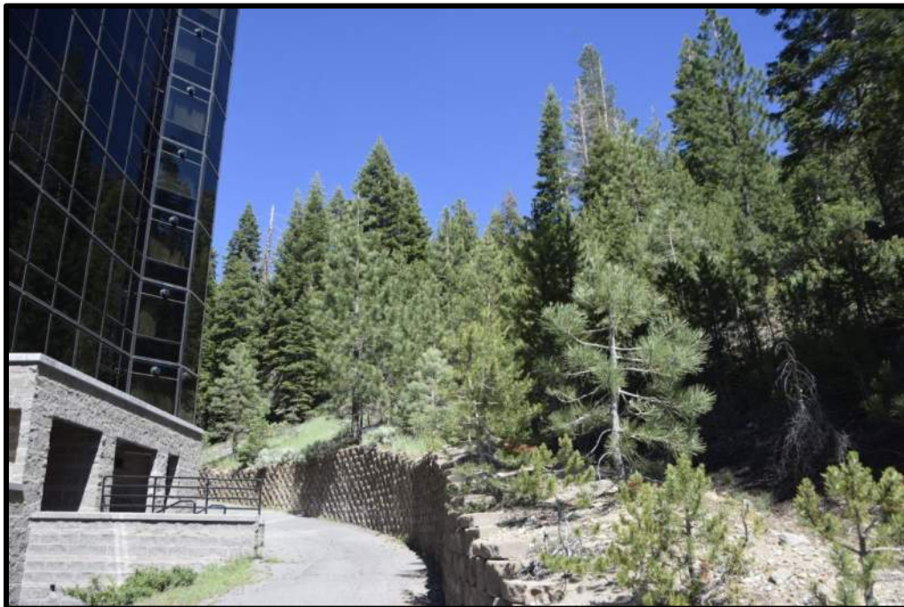
Figure 10: Pine thickets create a torching hazard adjacent to major infrastructure. This is not only a fire danger, but provides a bad example to the rest of community. This area should be heavily thinned within 150 feet of the buildings.
