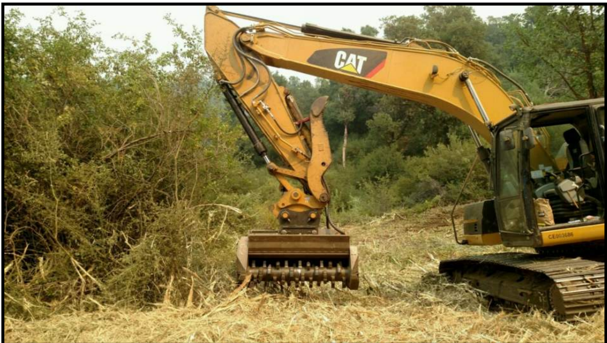
Figure 26: Excavator with masticating attachment.
