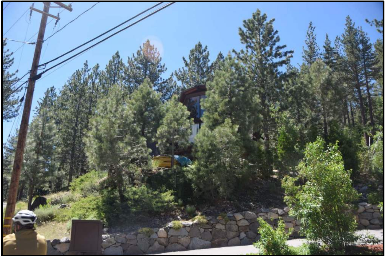
Figure 1: Heavy wildfire fuels adjacent to a structure
