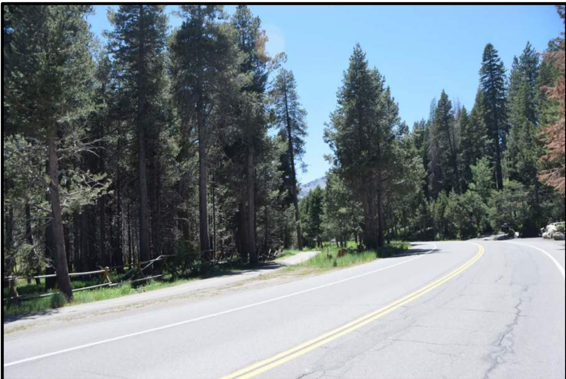
Figure 17: High hazard lodgepole thicket directly adjacent to the only road in and out of community. Lodgepole should be heavily thinned to remove ladder fuels.
